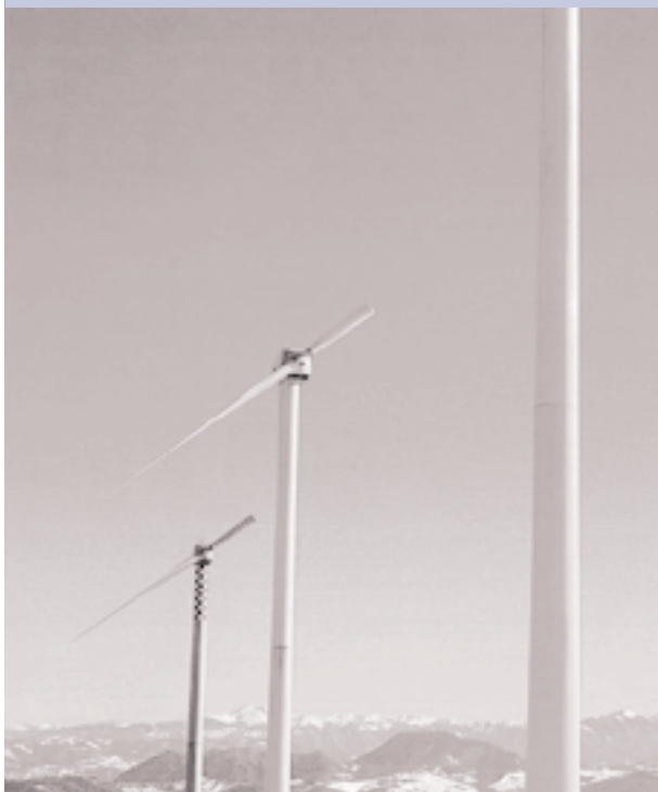
Figure 1.3: Single-Bladed Wind Turbine
