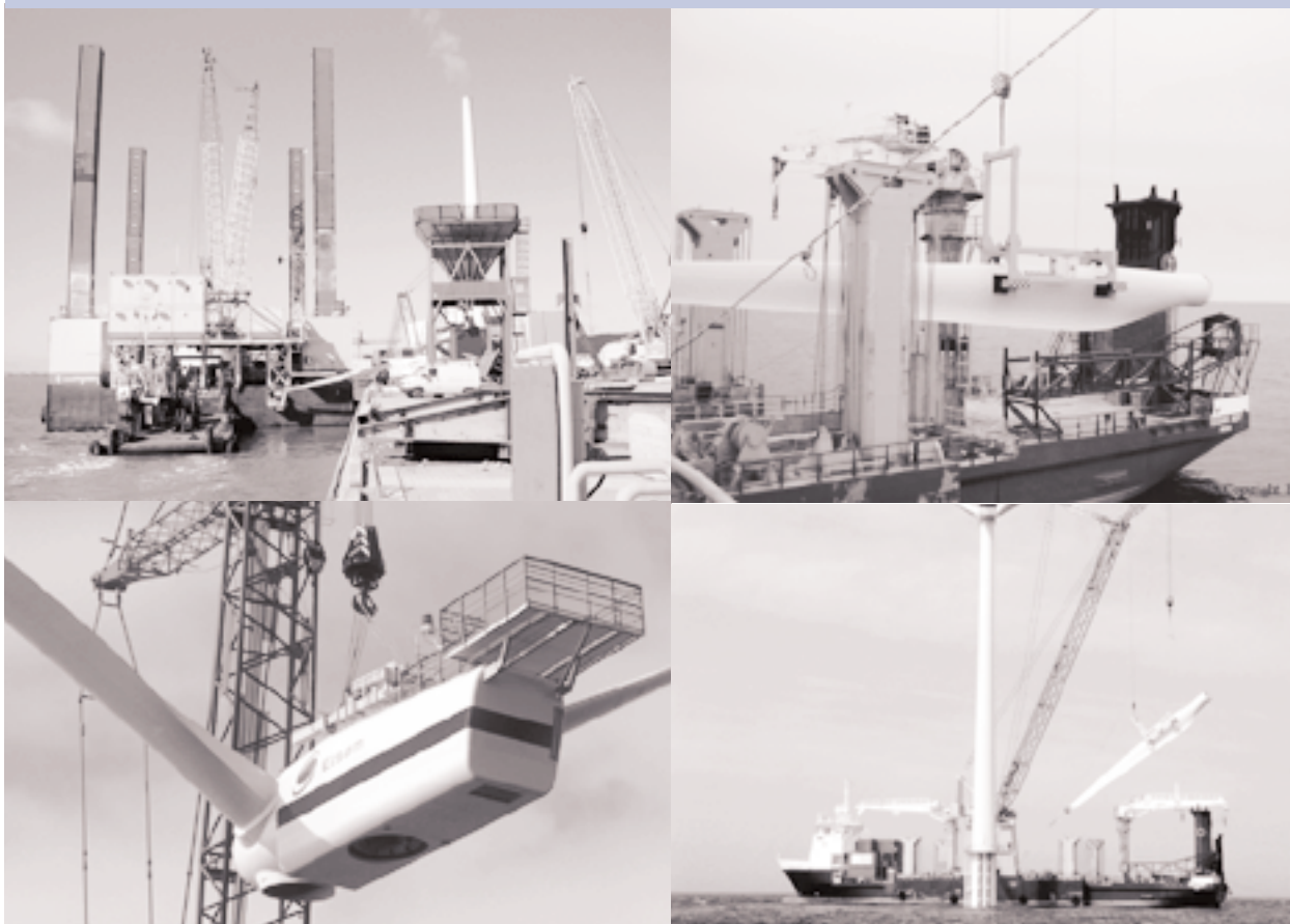
Figure 1.25: Erection of Offshore Wind Farms
