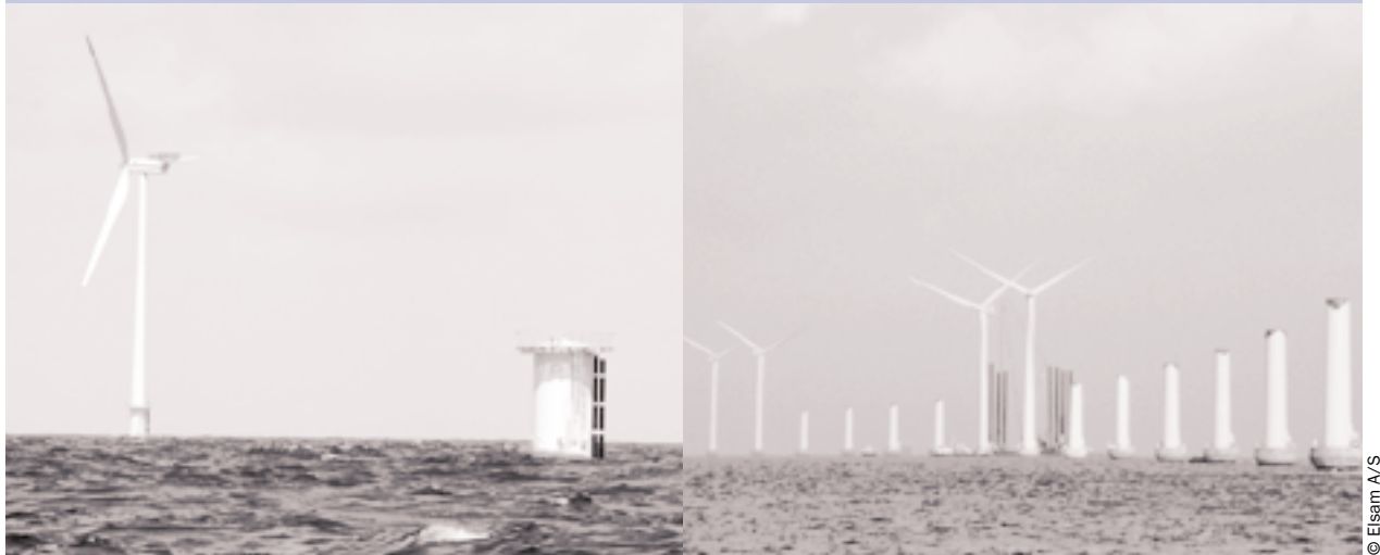
Figure 1.26: Erection of Offshore Wind Farms
